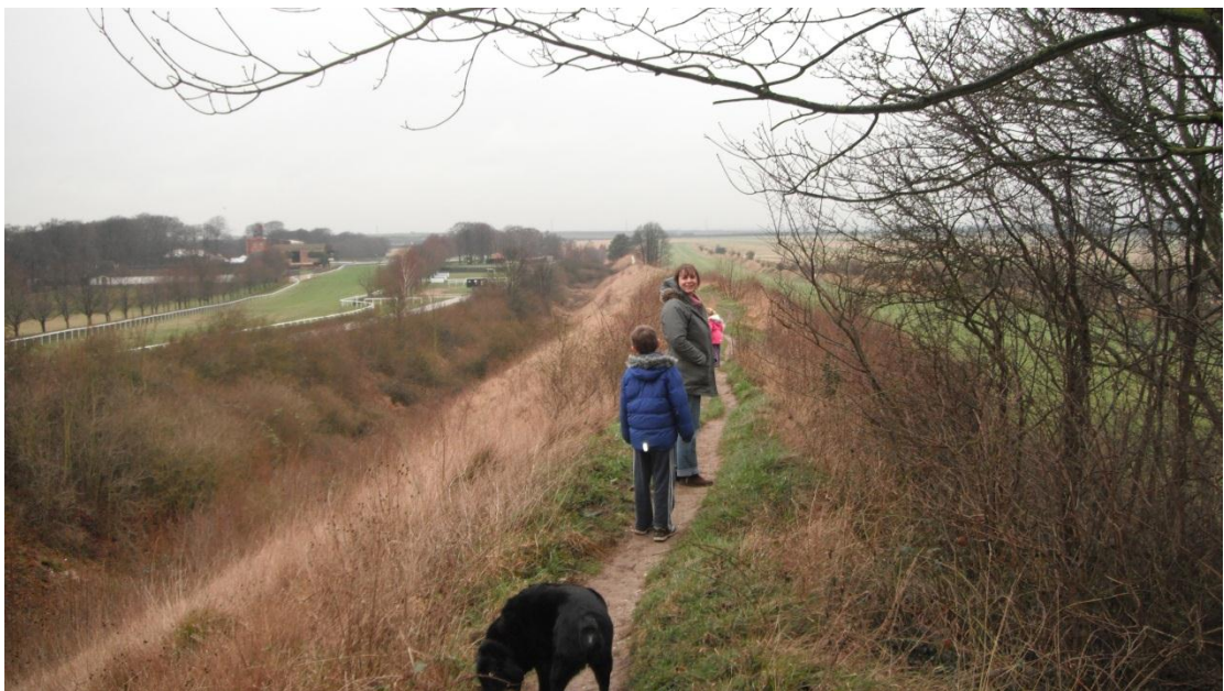
Figure 53 Devil's Ditch looking west
