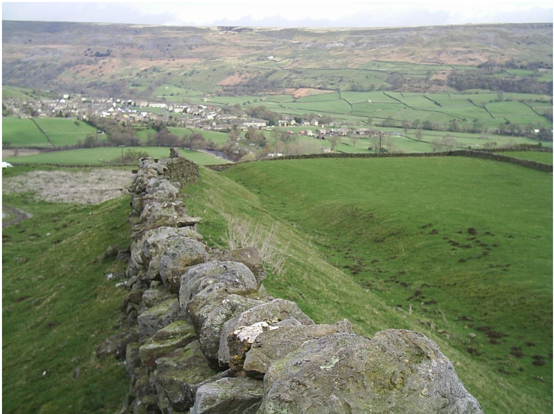
Figure 36 Looking north along the southern earthwork of the western group of the Swaledale Dykes
